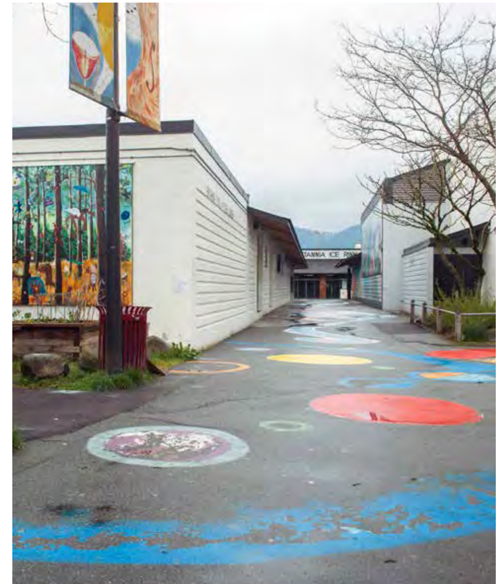
Britannia's facilities - arranged in a village layout - are nearing the end of their useful life.
